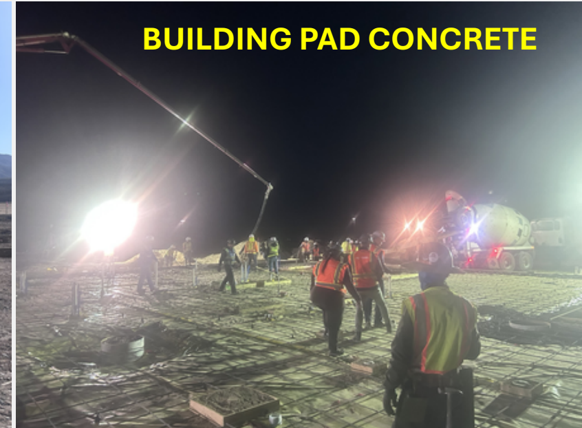
PLACING CONCTETE FOOTINGS
